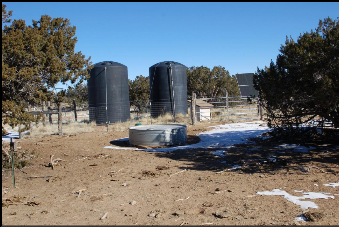
Livestock well with solar pump & storage tank
